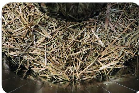
Evenly filled formwork
