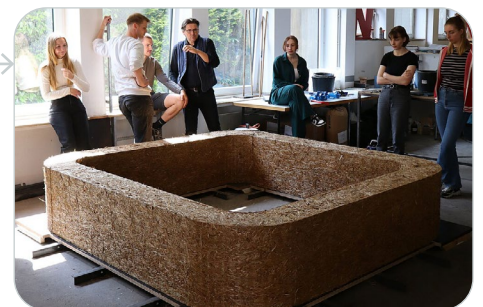
First frame removed from the formwork
