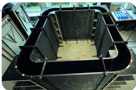
Frame formwork (1:1)
