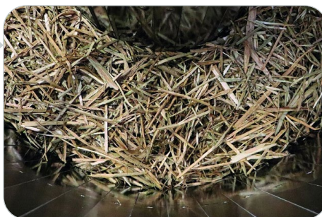
Evenly filled formwork
